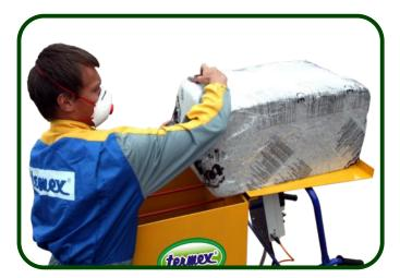
The insulation work itself is done easily by a team of two. One guides the blowing hose while the other one feeds the machine. The machine is controlled nice and easy with a remote control.
